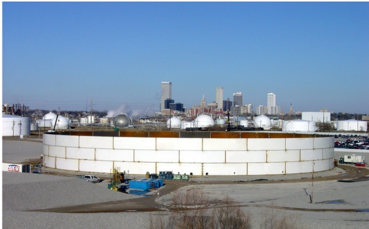
770,000 BBL Crude Tanks
