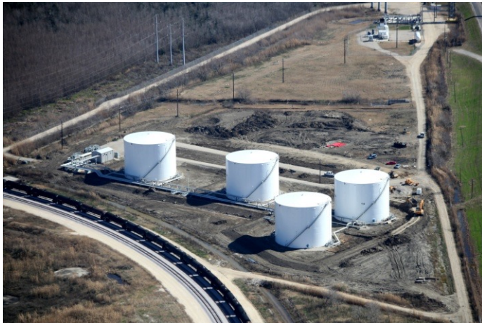
Foundations, Tanks & Painting 5 Months
