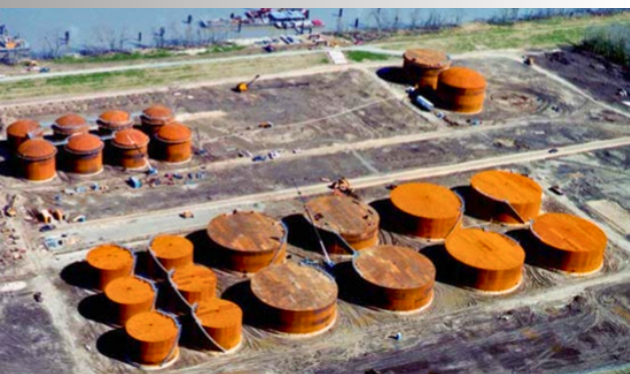
Civil, tanks, and painting 5 months, no overtime
