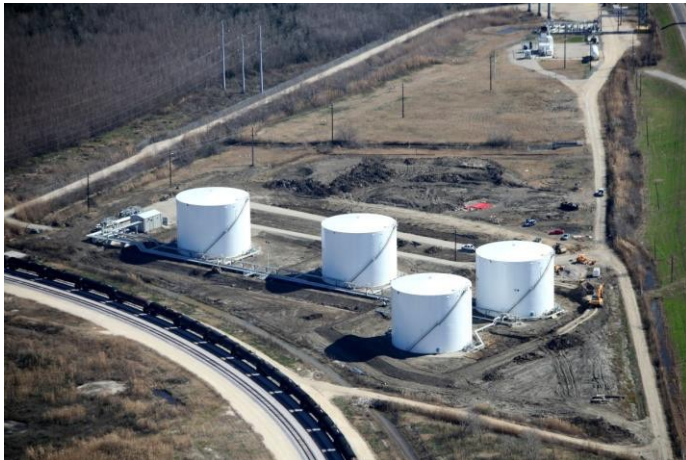
Foundations, Tanks, & Painting 5 Months
