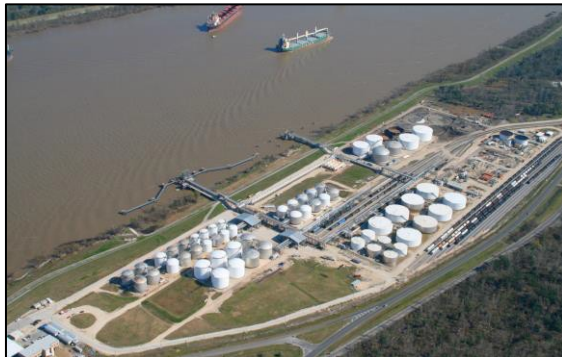
EPC for special chemical terminal – (58) various field erected tanks – carbon, stainless, IFR's and pressurized. – New Orleans, LA, USA
