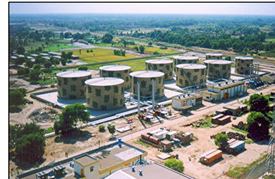
EPC for (10) – API-650 tanks from 40' diameter to 110' diameter – Multan, Pakistan
