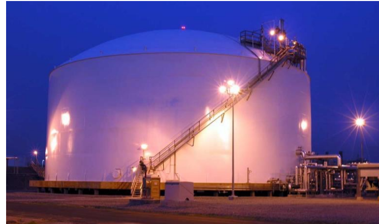
LPG/LNG Storage & Facilities
