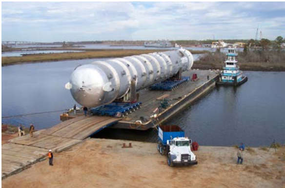
First Shipment from AT&V Waterfront Facility
