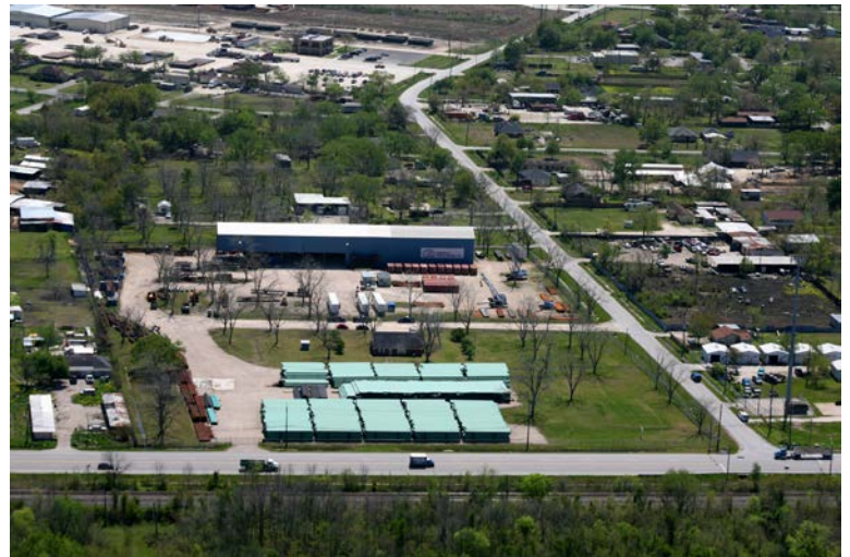
Houston Fabrication & Yard
